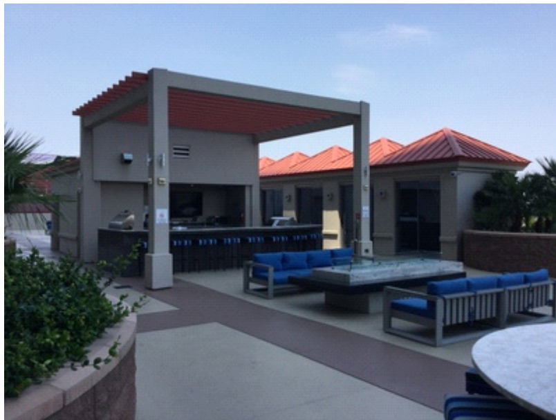
The Pool Components include Pool Re-surface, Re-seal, Heater, Pump, and Filter Replacement, Pool Furniture, Cabanas, Outdoor Kitchen and Spa Area. The remaining useful life of each Component is an estimation only.
