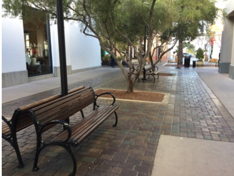
The Association is well maintained and in overall good condition.
