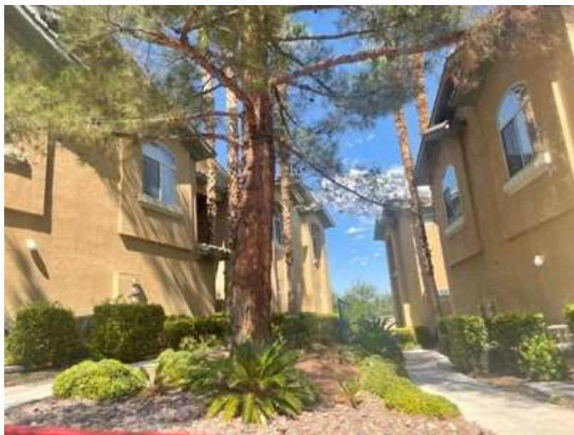
The Exterior of Homes Category includes the Tile Roof Underlayment Replacement, Exterior Painting and Stucco Repairs, Unit and Building Lighting, Building Signage and Paver Driveways. The Component Costs and Useful Life are an estimation only.
