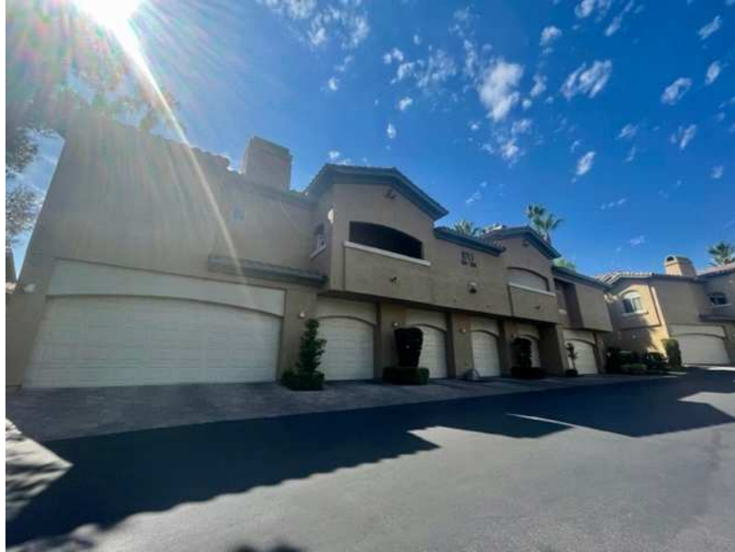
The Roof Replacement cost and estimated useful life was provided by PRS Roofing, Las Vegas, Nevada.
